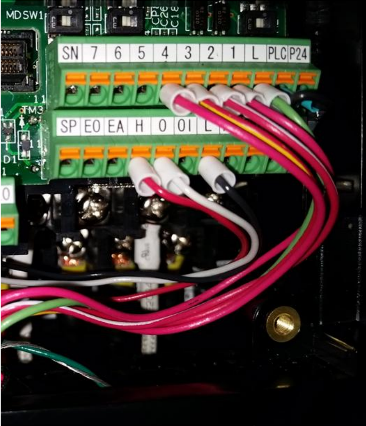
Use Star Grounding, Ground shields only at VFD end of cable.
