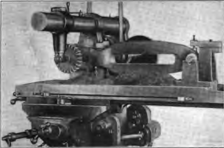
Fig. 19. Finishing End of Rocker-arm with Straddle Mill
